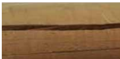
Splits, checks and cracks
